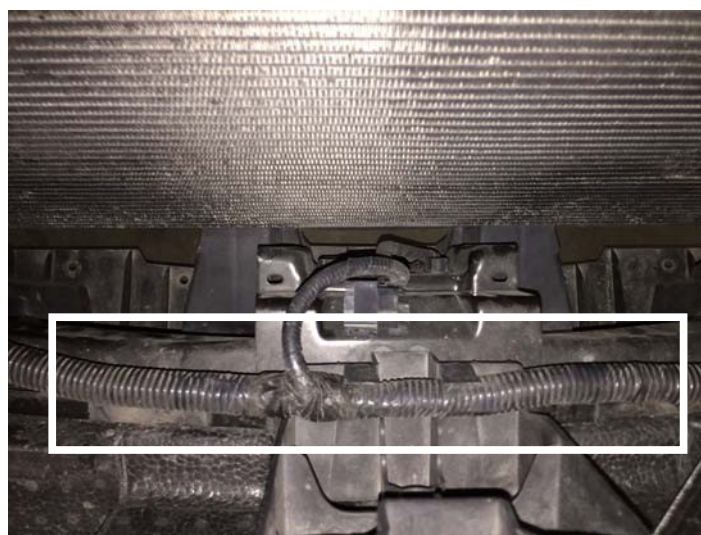
Move Wiring Harness
