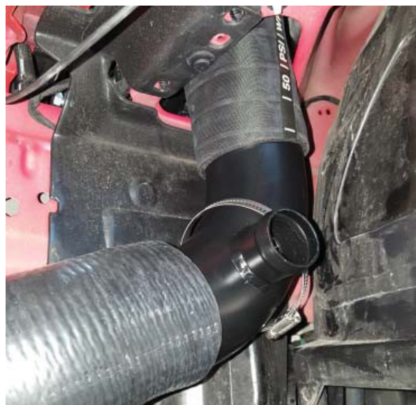
Surge Tube Installed
