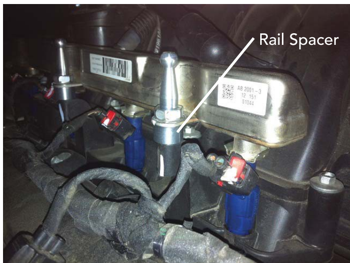
Fuel Rails Installed
