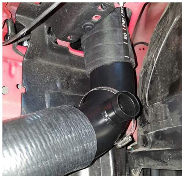
Surge Tube Installed
